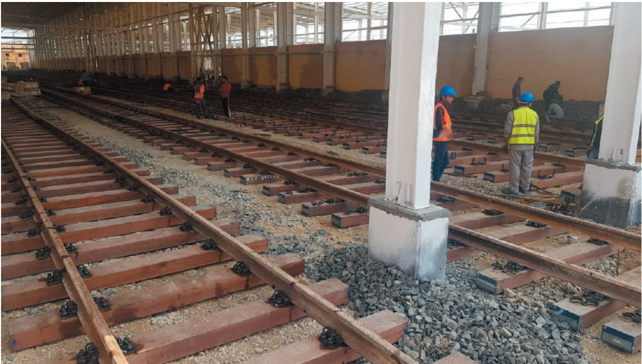
Sleepers made of Azobe in the Cairo metro in Egypt (photo Rail Europe)
