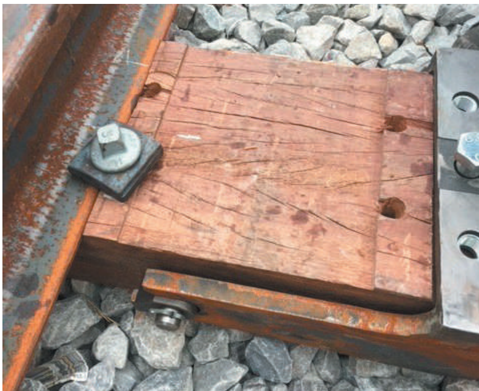
Detail of the assembly of an Azobe part (rail/tyre) for metro line no. 6 in Paris (photo: Rail Europe)
